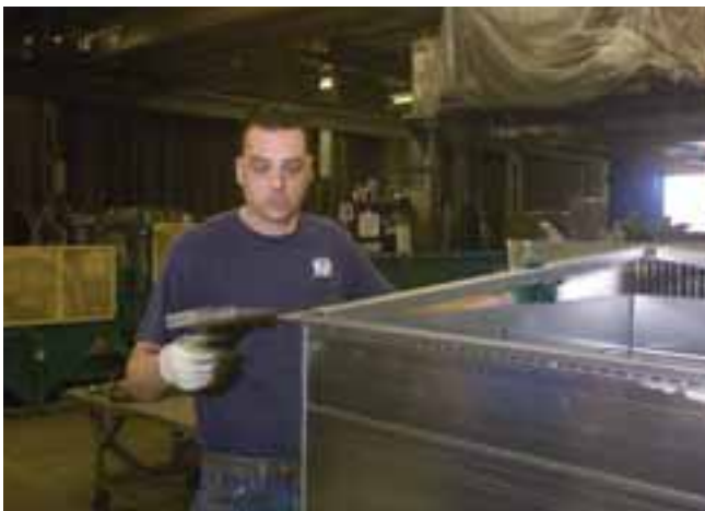
Vic Morset, F.E. Moran shop foreman, assembles corners and the Quick Flange frame onto a joint of riser ductwork going into the 10th floor mechanical room at Children’s Memorial Hospital in Chicago.
